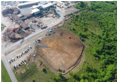
Pad before construction
