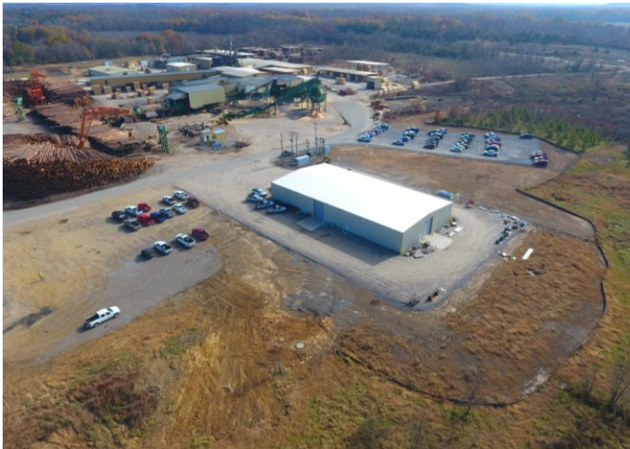
After with Maintenance Shop
